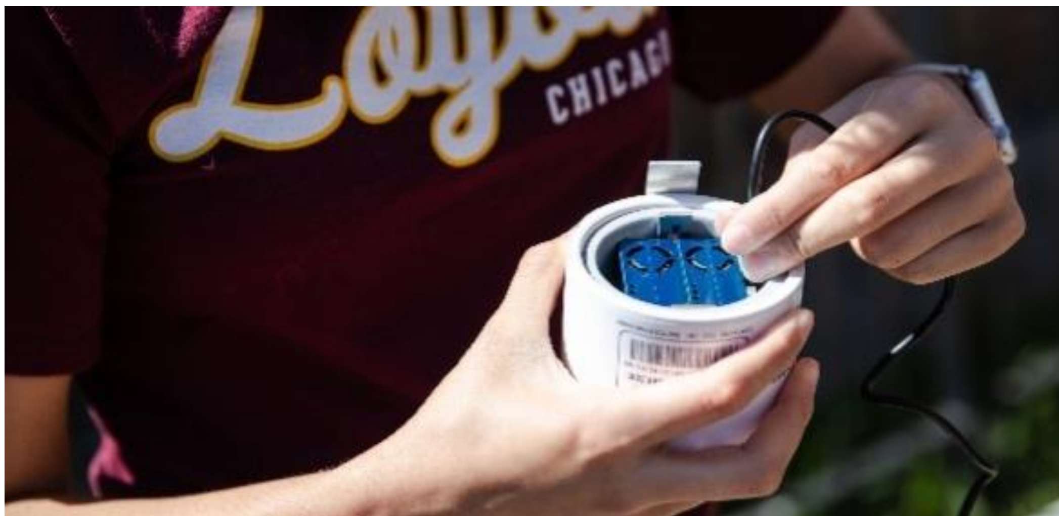
Fig 2. Loyola student from the CARE initiative installs a sensor
